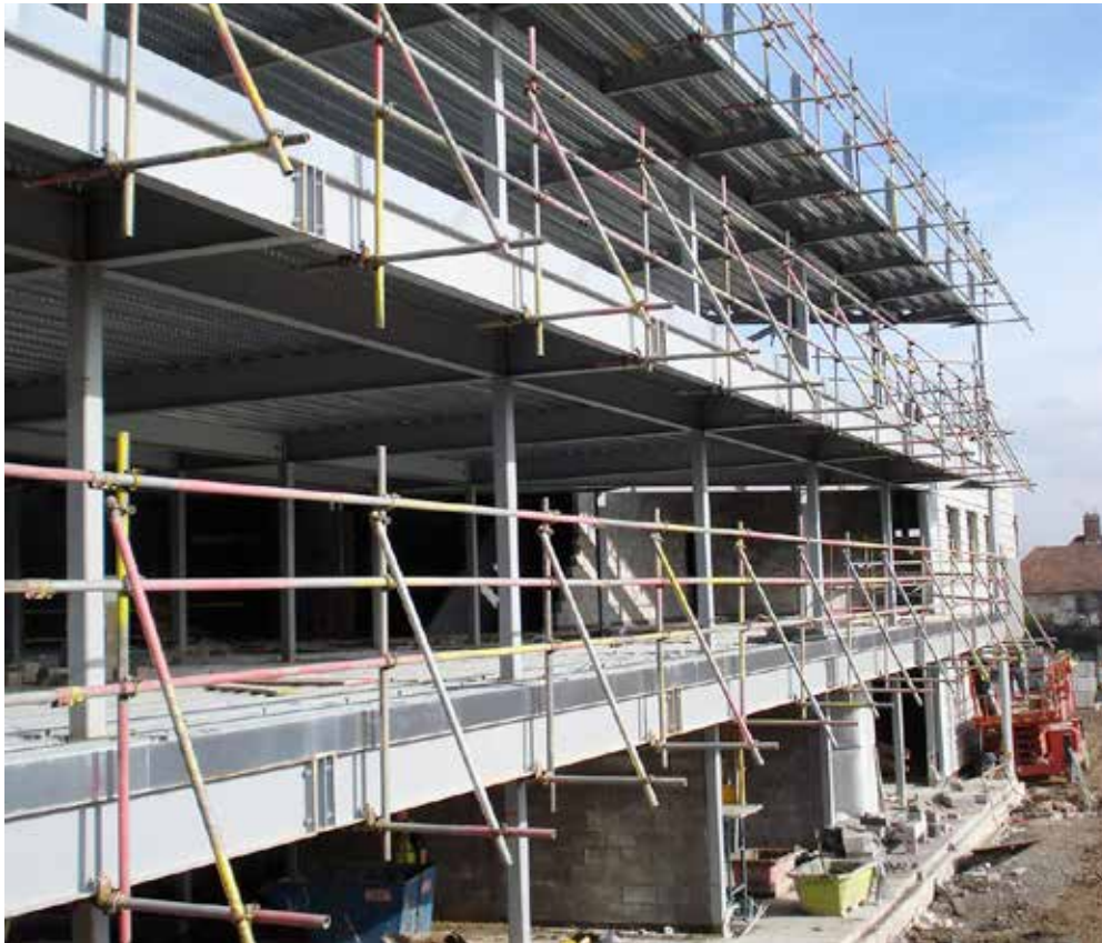
Knutton Road Studios during construction, February 2011. Photo: Yorkshire Artspace.
