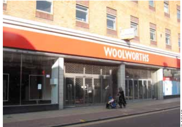
Former Woolworths Store, Peckham, London
