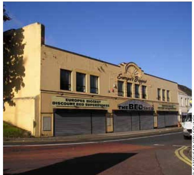
Former bed showroom awaiting conversion to artists' studios, Gateshead
